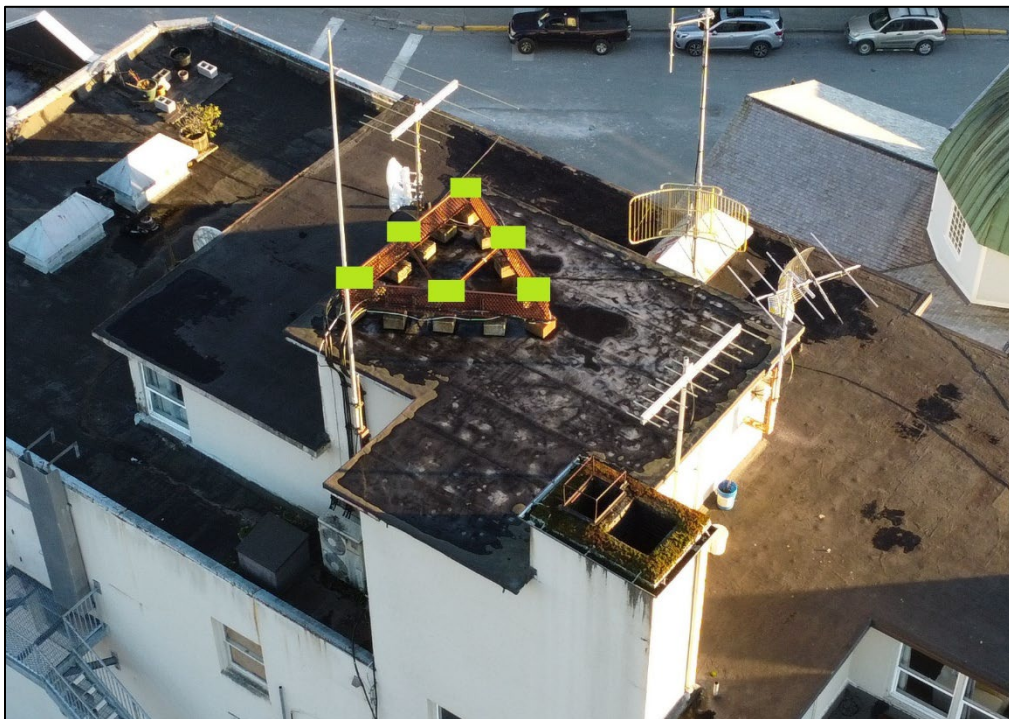
Photograph 9: Existing steel frame on penthouse with planned Star Link panels in green
