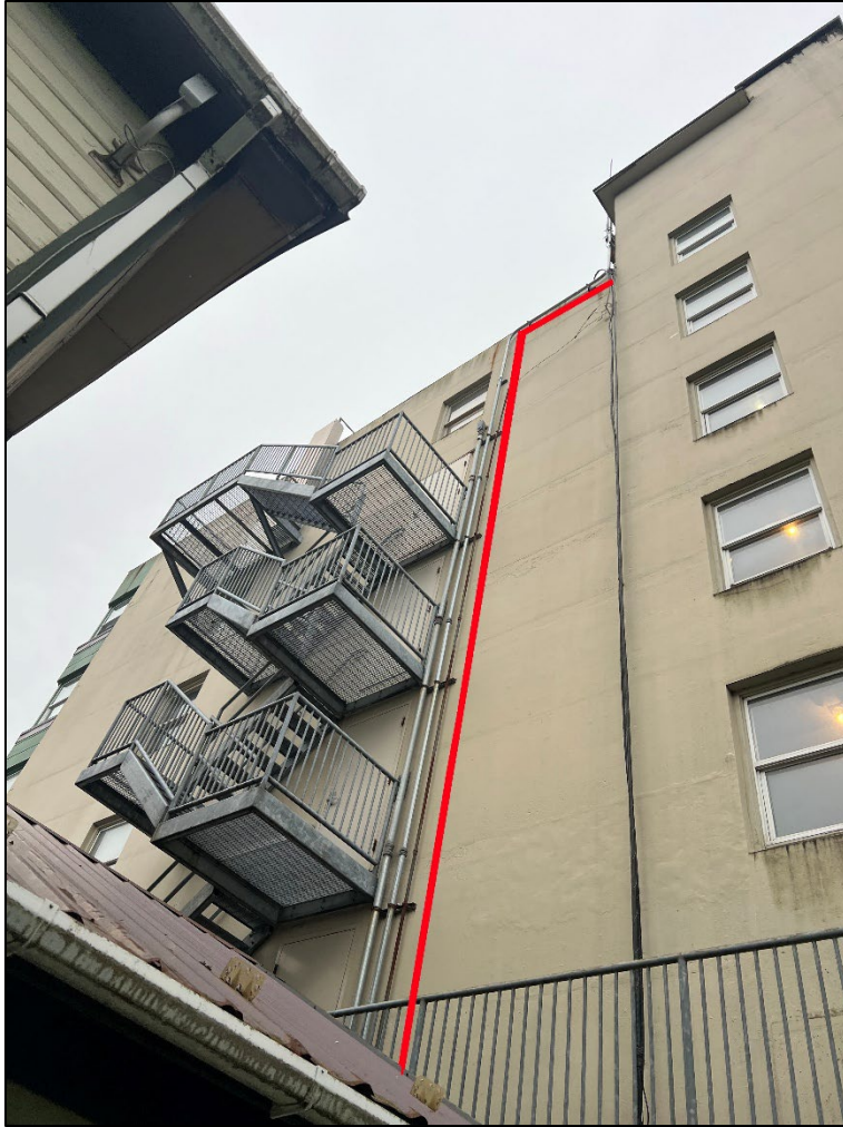
Photograph 10: Planned placement of new conduit down the northeast façade of the building
